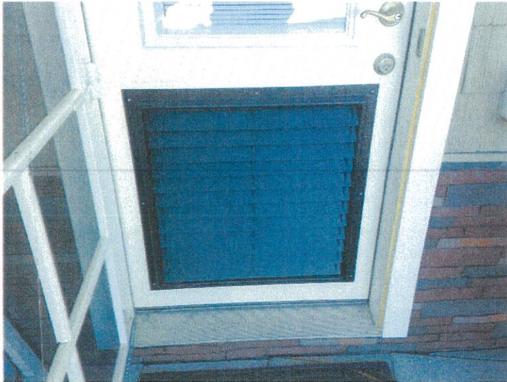
Garage Door With 24"x24" Louver Vent 17 Point Road 24"x24" Inside Garage Door
