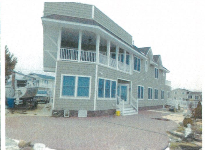
Rear With Louver Crawl Access
