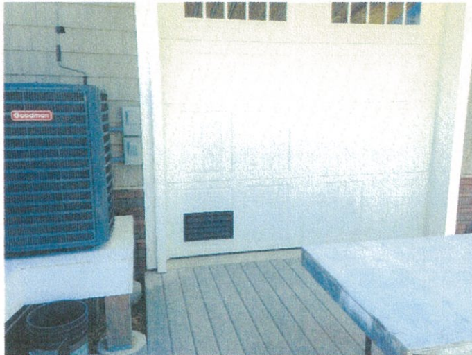
8"x16" Vent In Overhead Door 17 Point Road 8"x16" Vent Inside Overhead Door Pictures Taken 04/01/2014 & 04/30/2014
